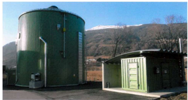
Anaerobic sludge stabilization and energy generation LIPP KomBio Reactor with CHP and condenser unit
