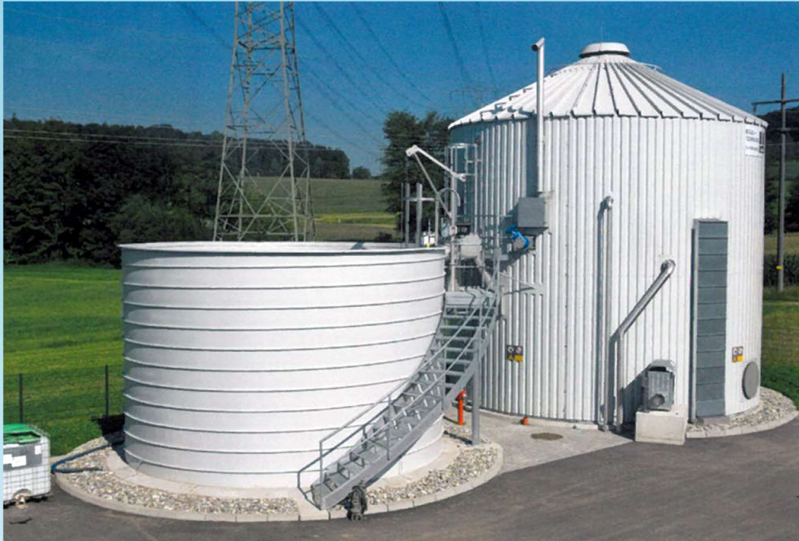
LIPP KomBio Reactor (60,000 gallons), sludge storage tank (35,000 gallons) on a municipal treatment plant
